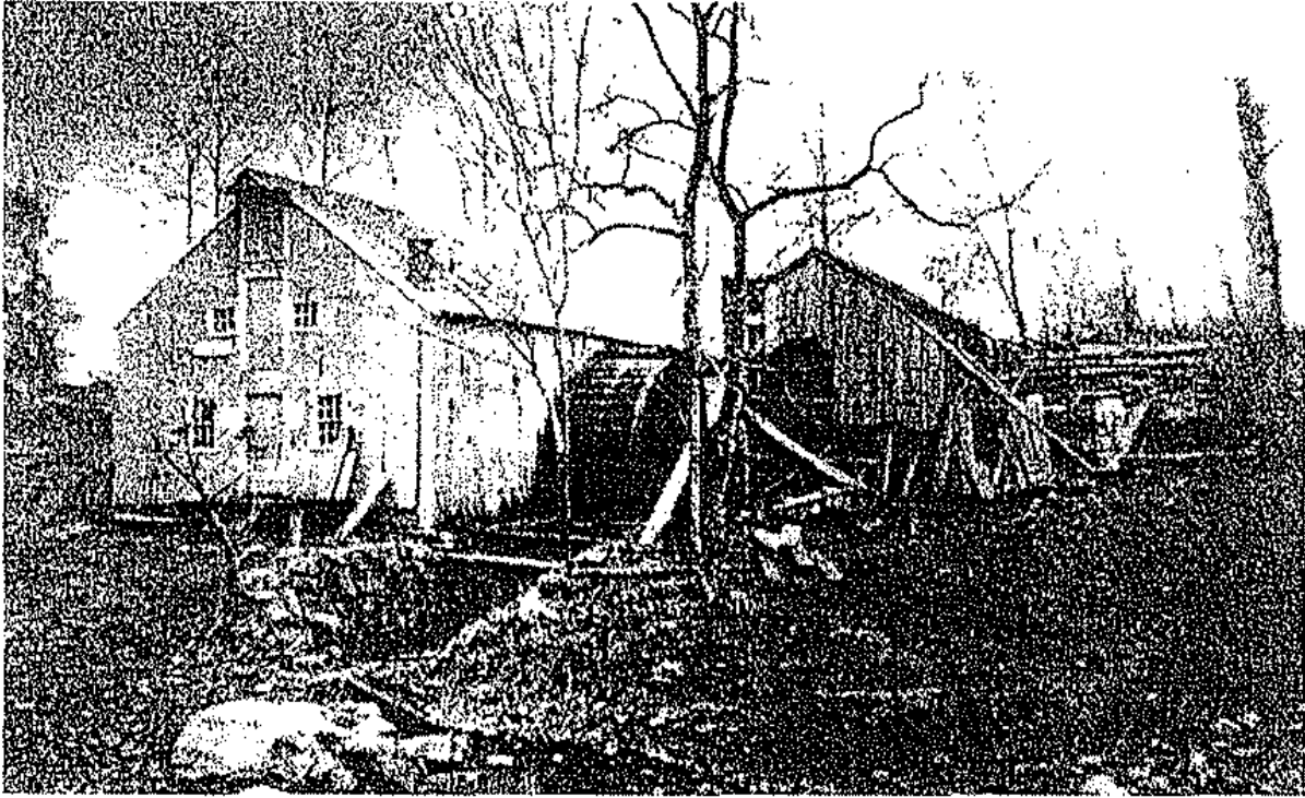
Wright's/Sands Mill before its demolition. 16
