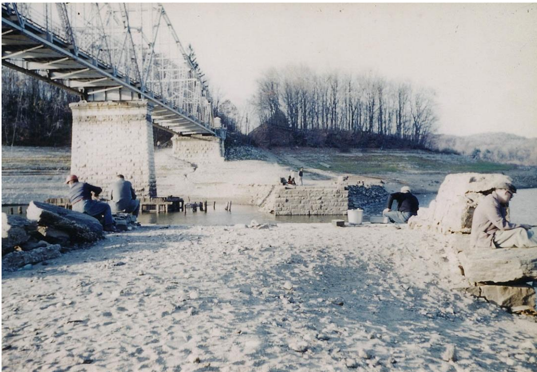
Pines Bridge crossing before the creation of the reservoir and the bridge on Route 100
